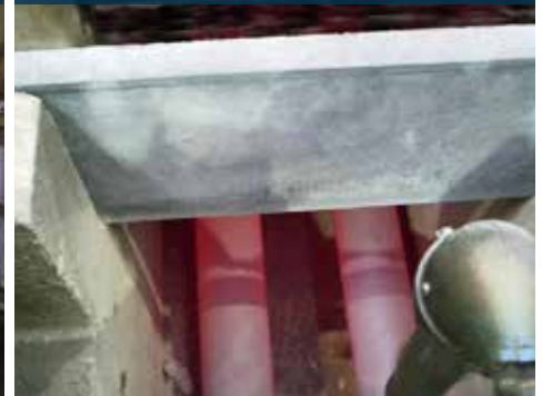
2,000KG immersion holding furnace
