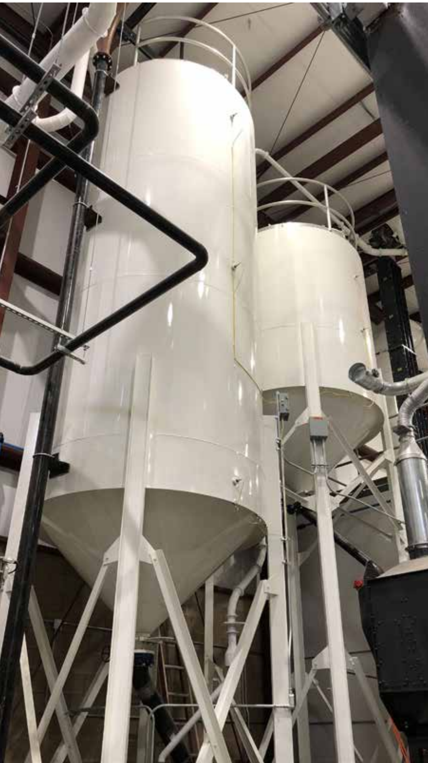
Bulk aggregate storage system
