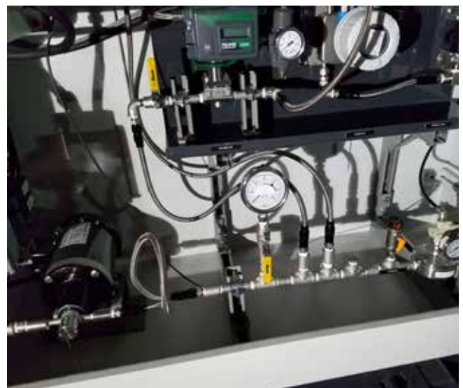
Mass flow pumping system
